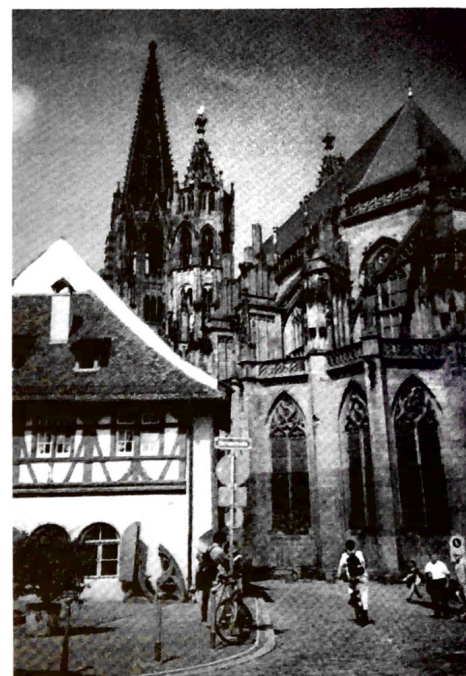
The Cathedral steeple will be covered in scaffolding while it is repaired
