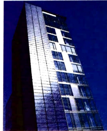
Photovoltaic panels at the railway station, one of Freiburg's many solar installations
